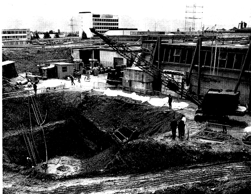
Excavation of the hole for the underground laboratory of the ISOLDE (Isotope Separator On-line Development) project. The project will use extracted proton beams from the 600 MeV synchro-cyclotron and the underground beam line from the SC is to be constructed during the present machine shutdown. (The SC building can be seen on the right.)
